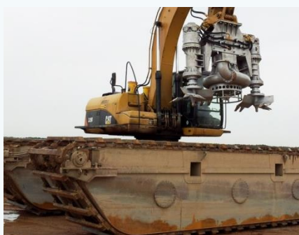
Pump installed on amphibious excavator
