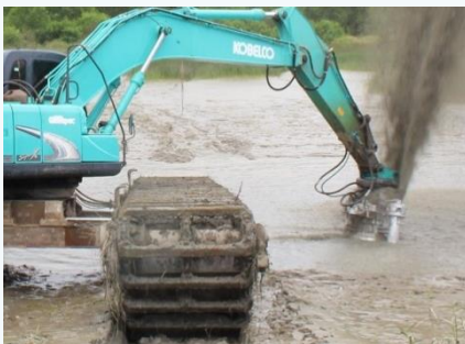
Amphibious excavator with Pump
